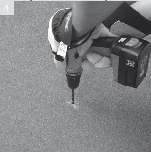
4 Drill 12mm holes in the three marked positions to a depth of 100mm to accommodate the bolt length, remove debris from holes
