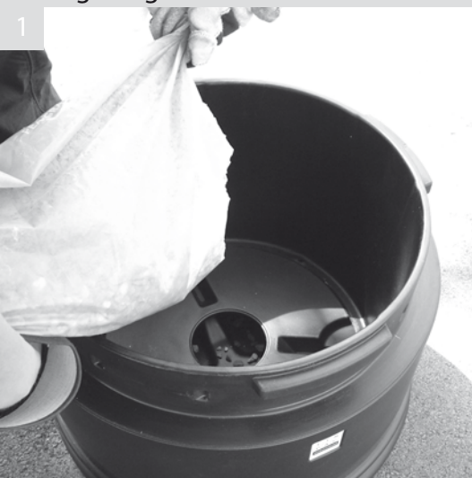
1 Remove cap from integral ballasting base and pour gravel into the center
