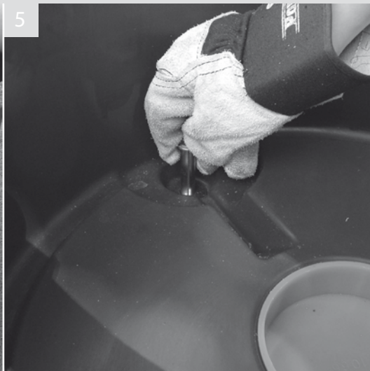
5 Re-position the base over the drilled holes. Add washers to bolts and push through moulded holes in base locating into drilled ground holes
